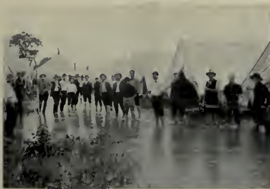
MAIN STREET DURING FLOOD
